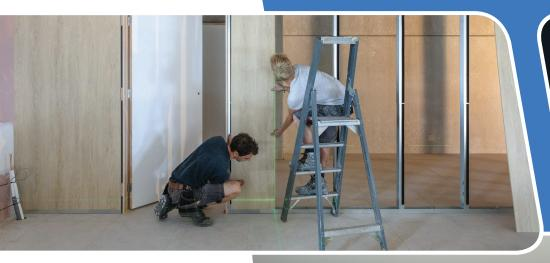
Clicwall is designed with a **click-together** mechanism, allowing it to be easily and quickly **installed** without the need for any special tools. **This can save** both time and money during the installation process.
